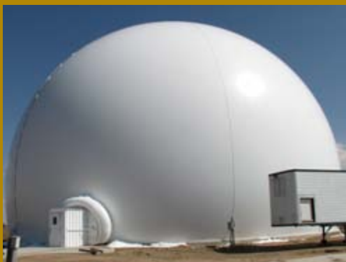
CSU-CHILL Radome and Airlock Entry
